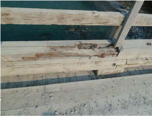
Figure 1-7: Guardrail rot.
