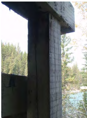
Figure 1-15: Downstream pier 1 post.
