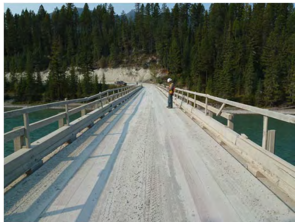
Figure 1-6: Bridge deck looking towards camp end.
