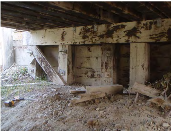
Figure 1-23: Woods end abutment.
