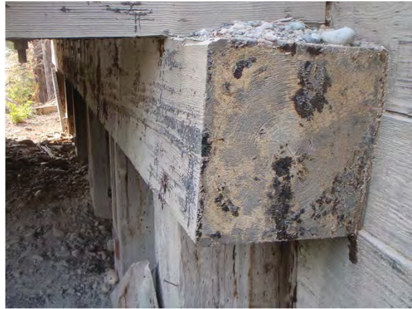
Figure 1-14: Camp end cap beam.
