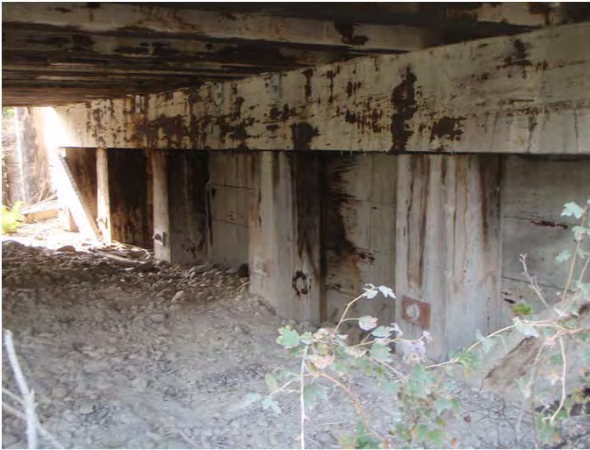
Figure 1-13: Camp end abutment.
