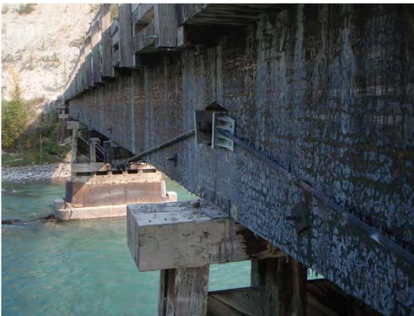
Figure 1-11: Upstream face of girders.
