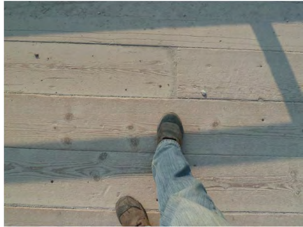
Figure 1-8: Typical deck condition.
